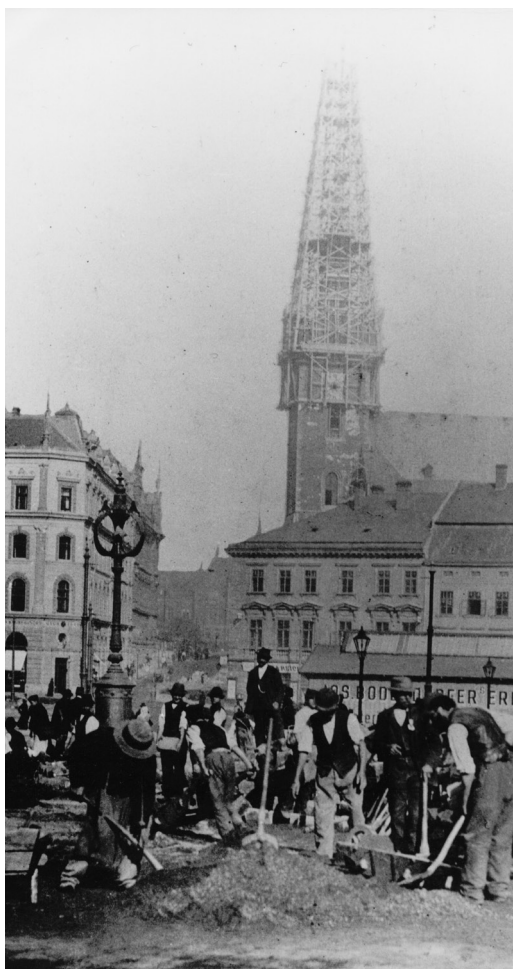
Brno c.1900. Tramway work to the fore, rebuilding at St James behind – site of an Antel clock.
