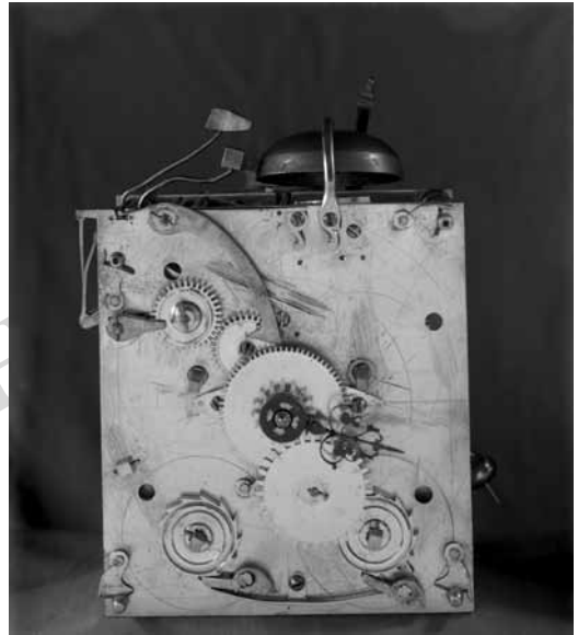
Fig. 11. Print from Negative 11 - Front Plate Movement View of a Thomas Tompion Unnumbered Table Clock.
