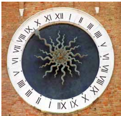
Fig. 4. The dial of the clock, with the central gilt sun and the 24 horary tiles, according to the hora italica tradition.
